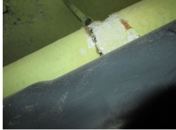
Figure 16 - Hanger with exposed parging in Room 011.
