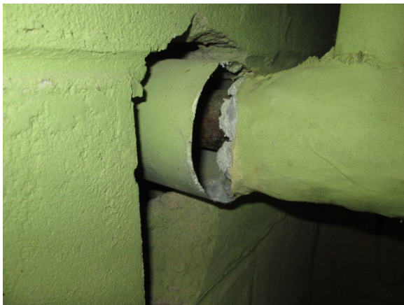
Figure 9 - The end of the pipe entering the wall cavity in Room 006 (under stairs storage) has exposed parging.
