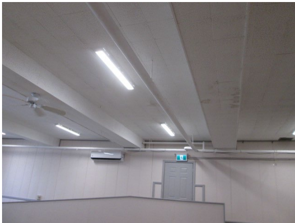
Figure 2 - Bulkheads throughout the basement level, including Room 001 shown, may enclose additional pipe parging fittings.
