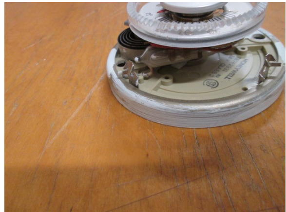
Figure 29 - A mercury vial can be seen in this uninstalled thermostat observed in the storage under the stairs in Room 006. See Figure 30.
