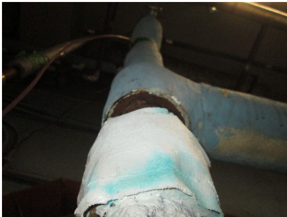
Figure 14 - This fitting in Room 010 is partially covered, but some exposed parging remains.
